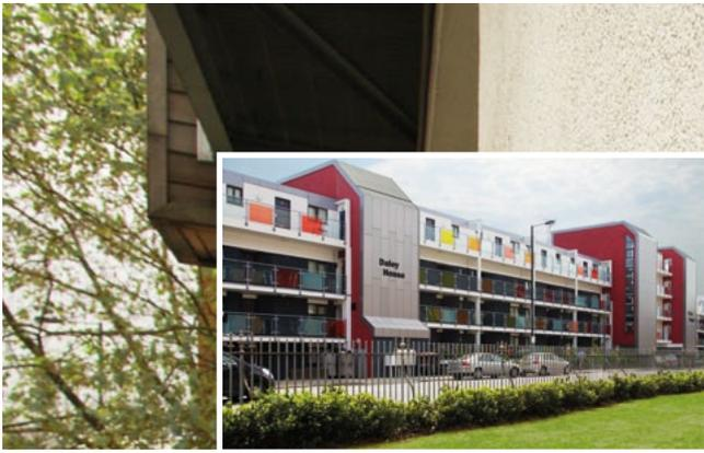
Prefabricated pods have been craned into position over the older 1970s blocks, creating a fourth floor of flats
